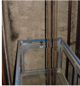
Asbestos on hoistway walls – risk of severe health effects if put in contact or removed without precautions.
