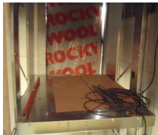
Risk of falling from inside the car when exposed to a fall hazard
